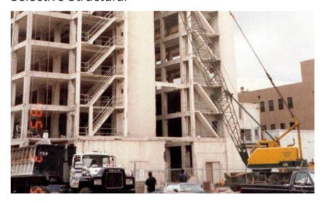
Structural improvements & modifications are relatively expensive design variables; therefore, owners incorporate the existing structural members whenever possible. The challenge is to "surgically" remove the necessary structural components without compromising the safety of the workers or the structure's integrity.
