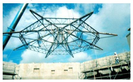
The reverse of the constructing sequence. Often necessary due to extenuating circumstances such as other improvements, proximity of occupants; and/or structural integrity issues.
